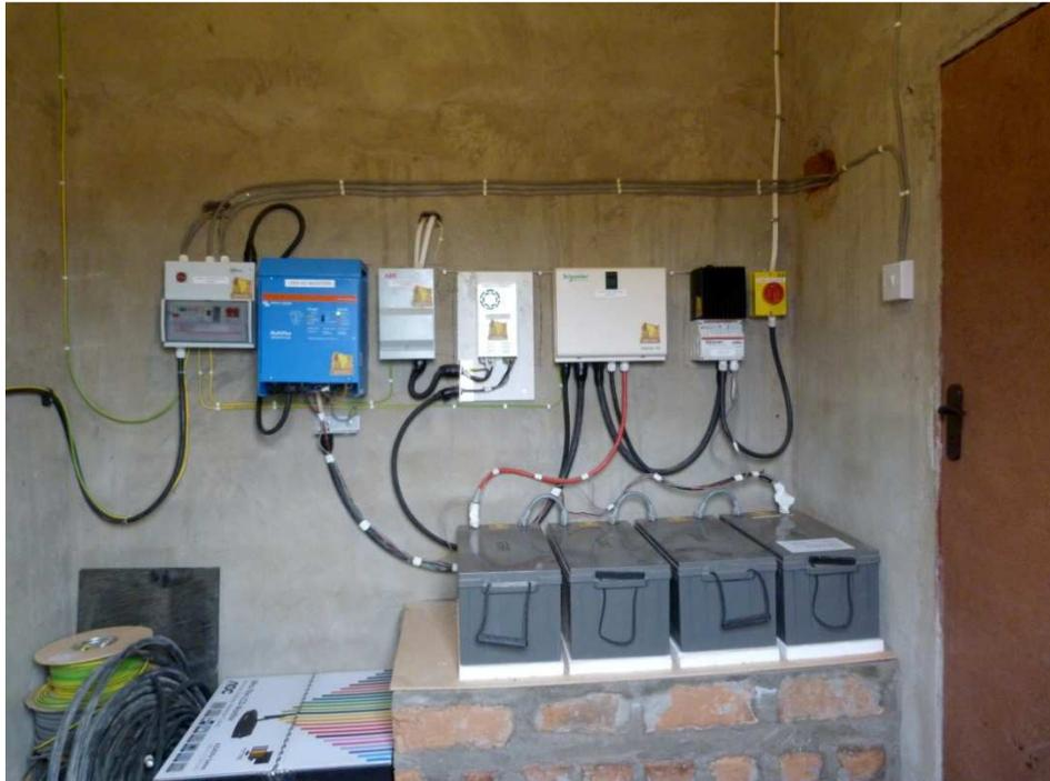
**Figure 3 - Switchroom equipment. Wall mounted equipment from left to right; 230V-AC distribution board (wylex), 3kVA Inverter, 12V-DC distribution board, 48V-DC:12V-DC converter, 48V-DC distribution board (schneider), Maximum power point tracker (Morningstar), solar panel isolator.**
